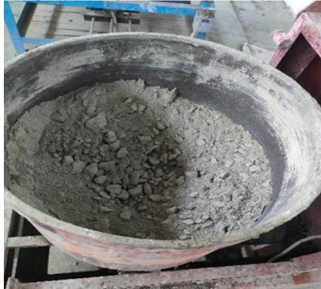
Figure 2.1: Concrete Mixing Process
