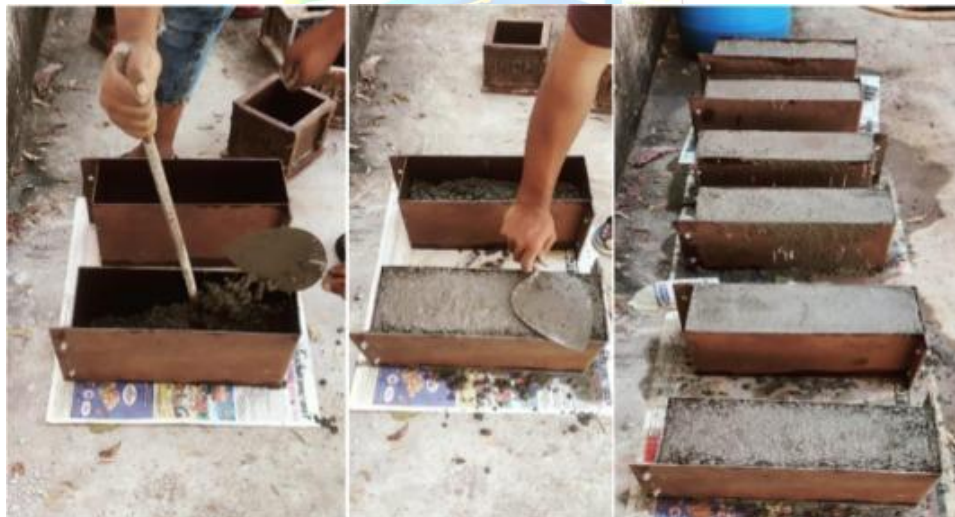
Figure 2.2: Casting of Paver Blocks
