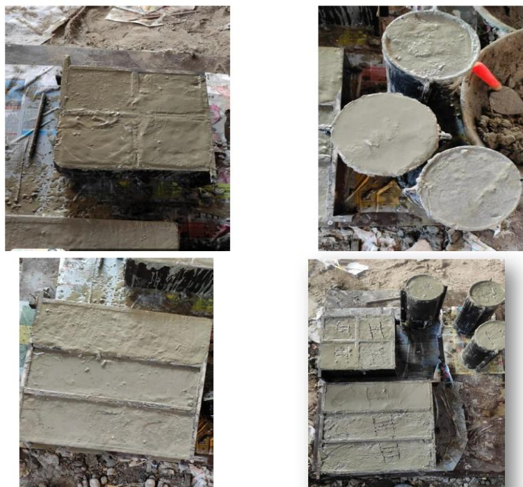
Figure 3.1: Concrete Casting Process
