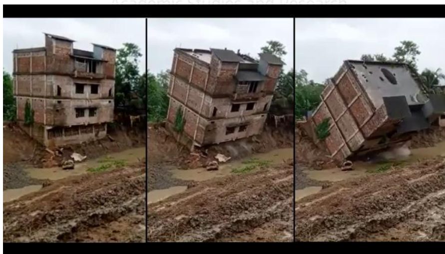
Figure 1.2: Earthquake Effect on Building on Sloping Ground
