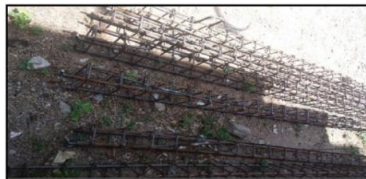
6(c) Reinforcement Cage
