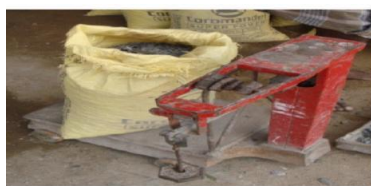
6(a) Batching of Materials
