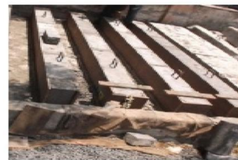
6(f) De moulding Under Progress
